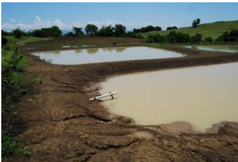
Fig. 4: Ponds lacking anti-erosion measures, PNLCH, Savanne Baptiste area, FAO, Renald and Maxi
